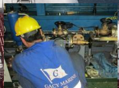
Flow meter installation
