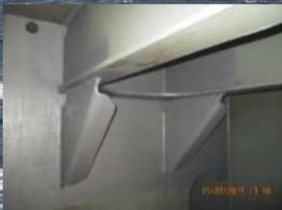
BWT damage repair
