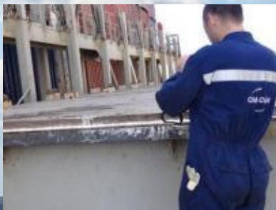
Hatch cover repair
