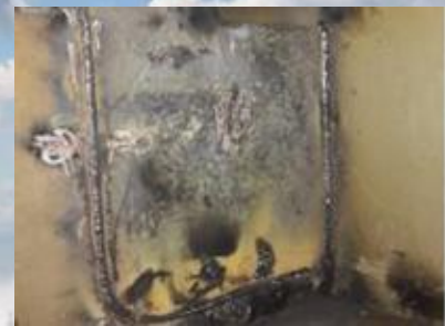
Void space repair
