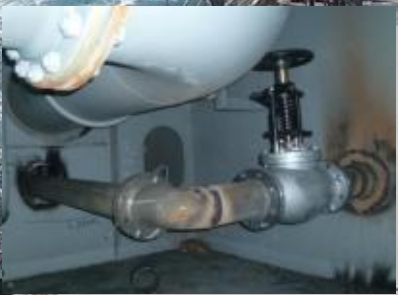
Fuel piping modification
