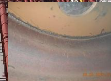
Tube sheet welding
