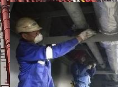
Sewage piping modification
