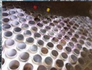
Tubes replacement-Water side
