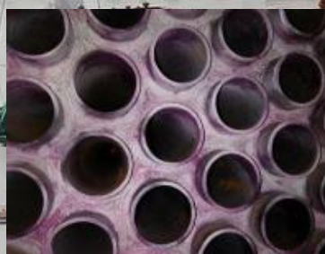
Tubes replacement-Water side
