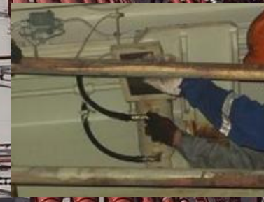
Ramp Hyd. Hose fabrication
