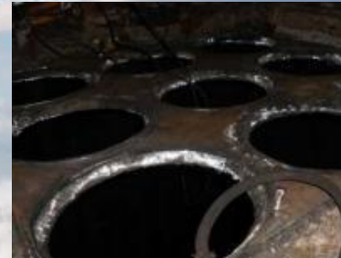
Tube sheet repair
