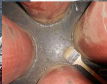
Welding of the tubes
