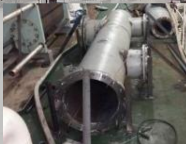
Sea water pipe fabrication
