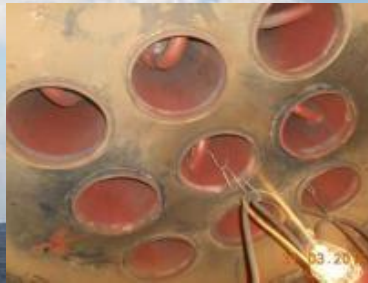
Tubes replacement-Fire side
