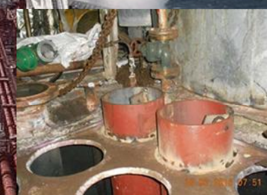
Welding of the tubes
