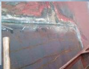
Hull shell plate repair
