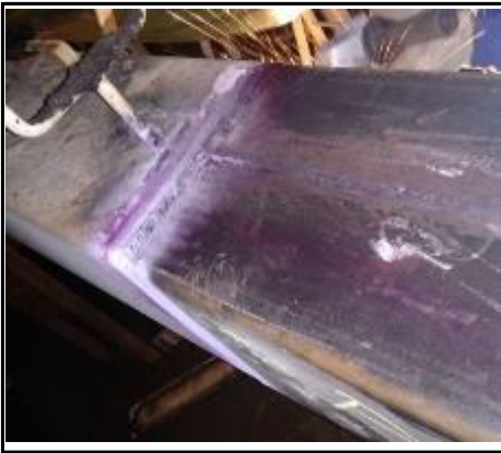
PT test after UT test under the witness of ABS surveyor
