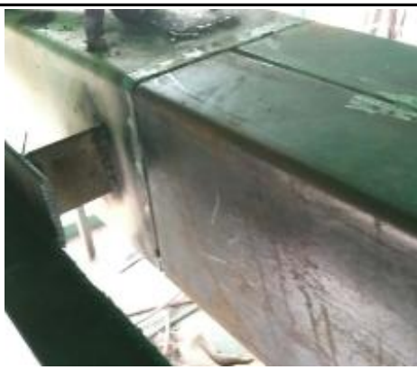
Fitted up the new material
