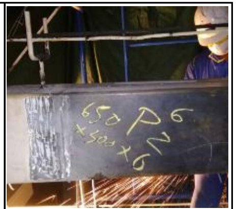
UT test after welding under the witness of ABS surveyor
