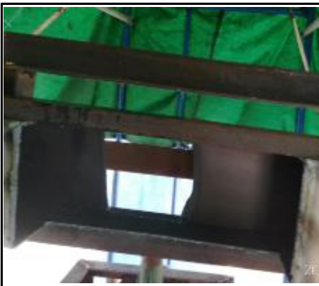
Cut the damaged area(complete by two times)
